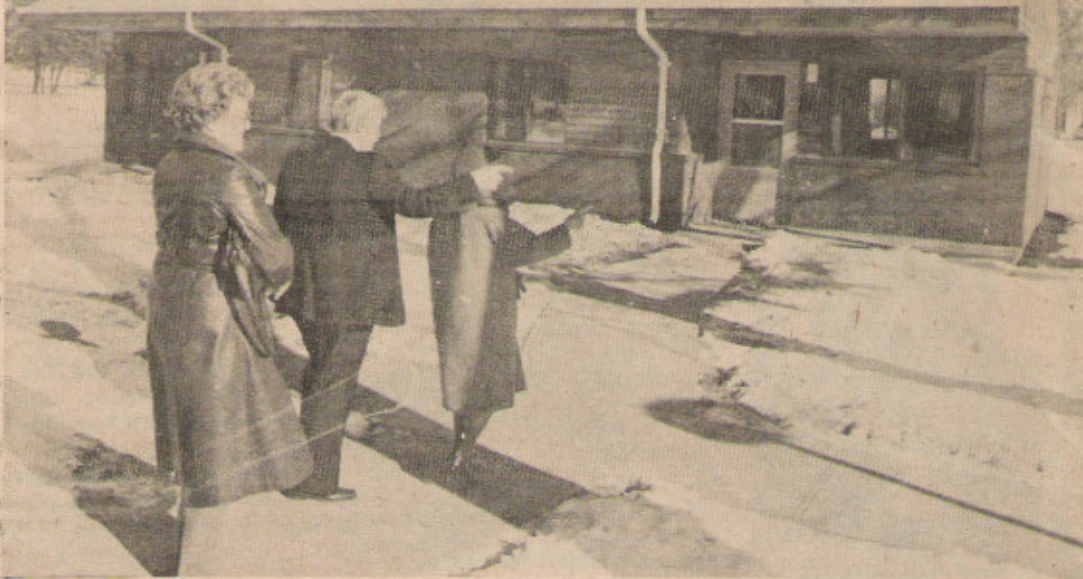
HORDVILLE HOUSING AUTHORITY chairman Roger Gustafson takes Lindenwood visitors on a tour of the low income housing development in Hordville during the facilities grand opening on Sunday. The eight-apartment duplex-designed complex is ready for occupancy, with several residents already moved into their new homes. — News-Register Photo
