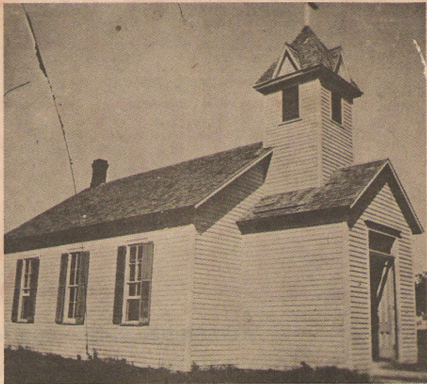
FRIDHEM LUTHERAN CHURCH around 1906 was located in Section 21, Township 13, Range 5 which is the Hordville community. There is an entrance room with a belfry topped by a cross and shutters on the windows. Plainsman Museum collection picture is courtesy of the Veburg family in Hordville. —News-Register Reproduction.
